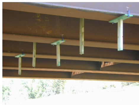
Figure 6: Rulers installed on steel girders to measure deflection.
