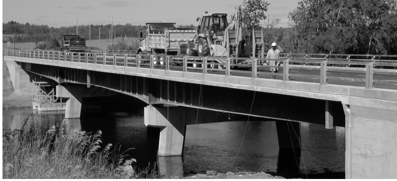
Figure 8: Magog Bridge – on Highway 55 North, Québec, Canada
